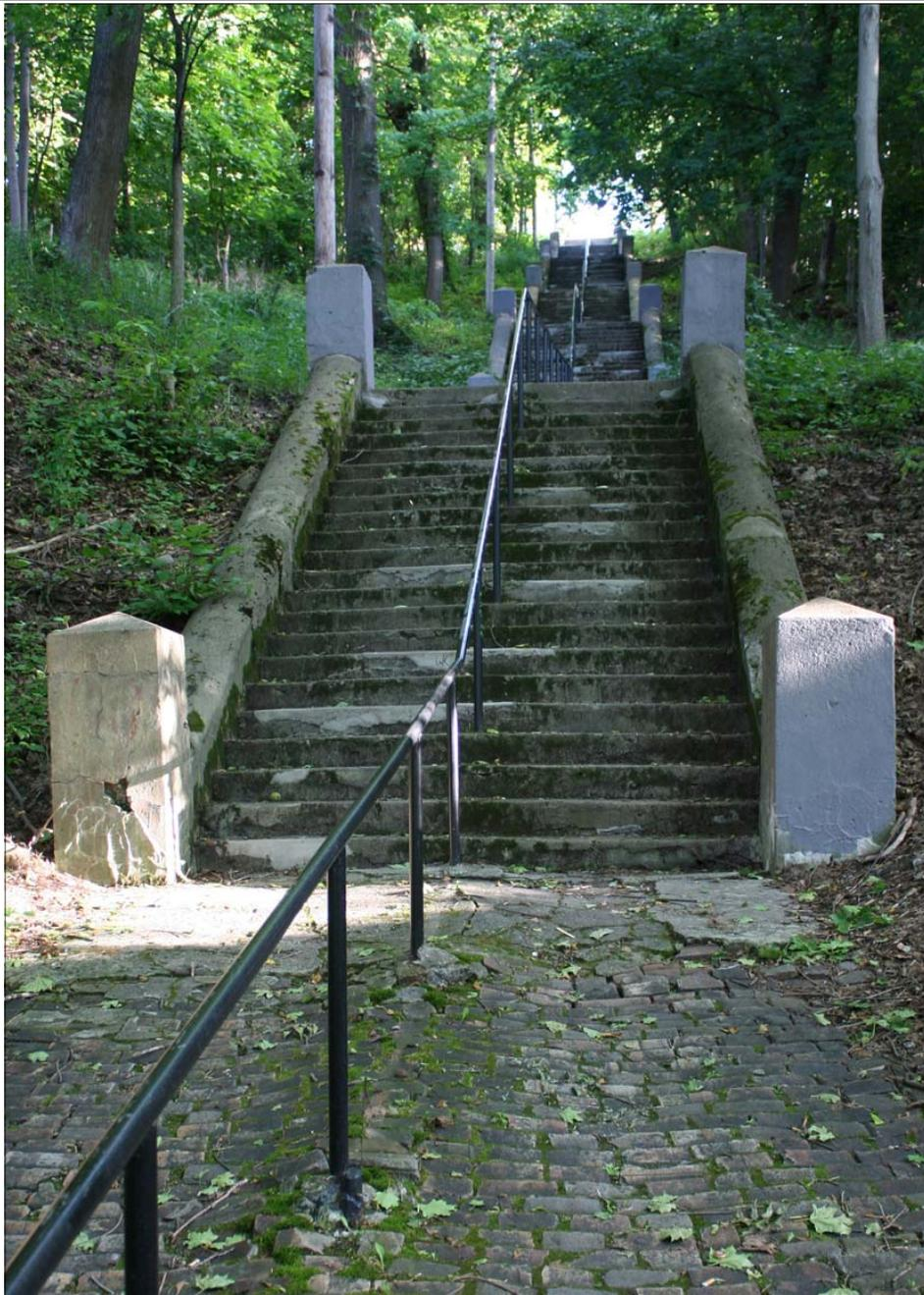
SEUNA led efforts last year to address the poor condition of the Westminster Steps. As a result, the city replaced the center handrail from top to bottom and many of the concrete steps have been repaired. Obviously, there is still work to be done.
